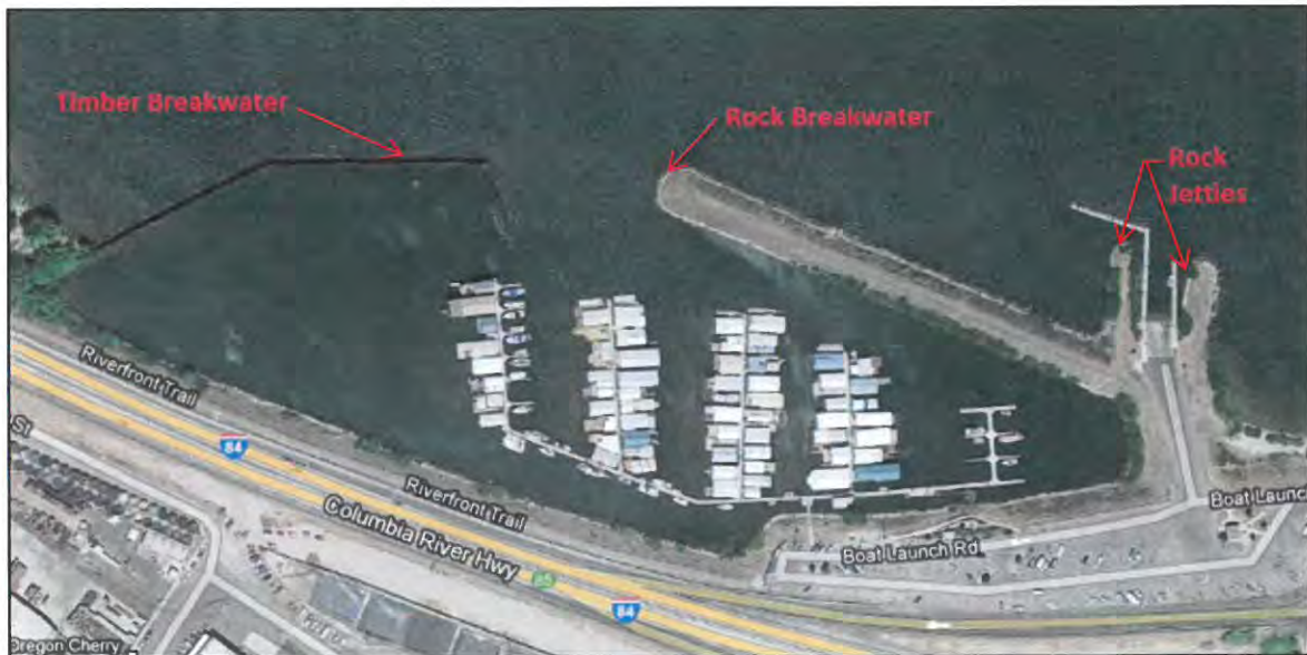
Figure 2. Aerial of Marina and Boat Launch
