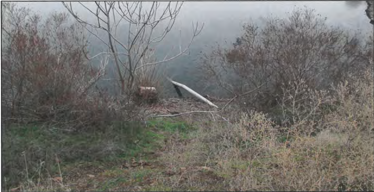
Figure 13. Water Line to the Marina
