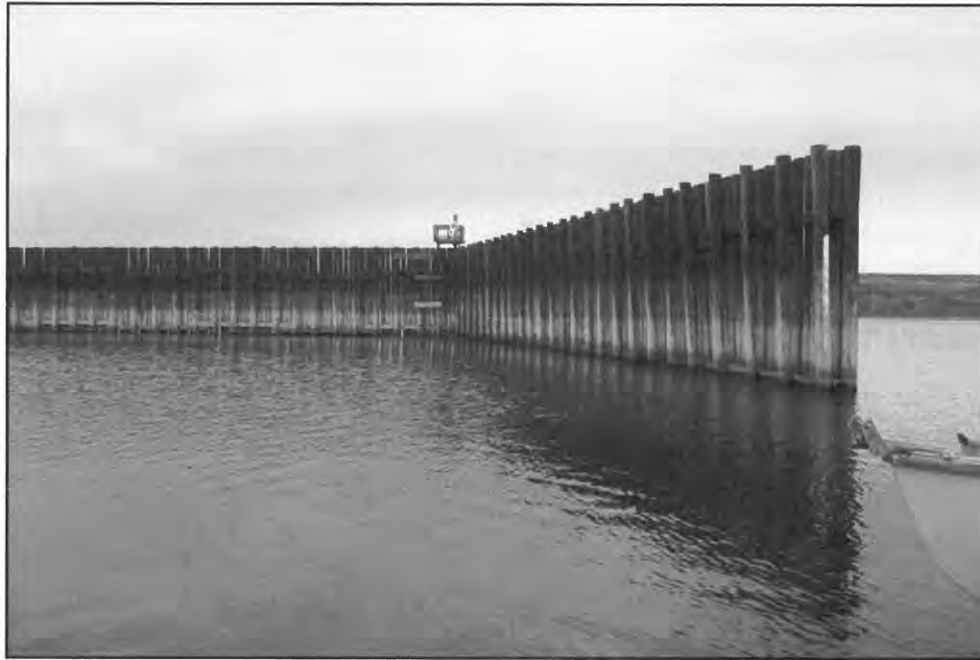
Figure 3. Timber Pile Breakwater
