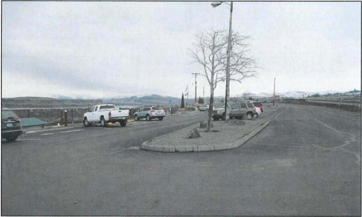
Figure 14. Marina Parking Lot
