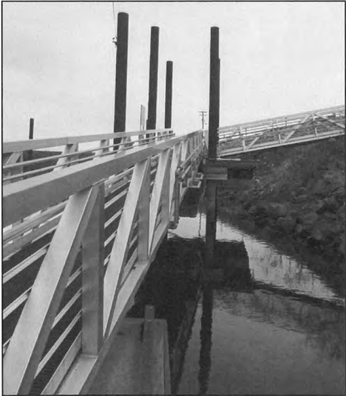
Figure 5. ADA Accessible Ramp
