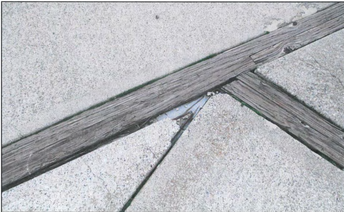
Figure 7. Concrete Spalls on Floating Dock
