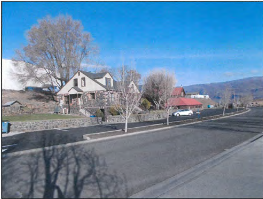
Figure 2 - Port of The Dalles Office Facilities
